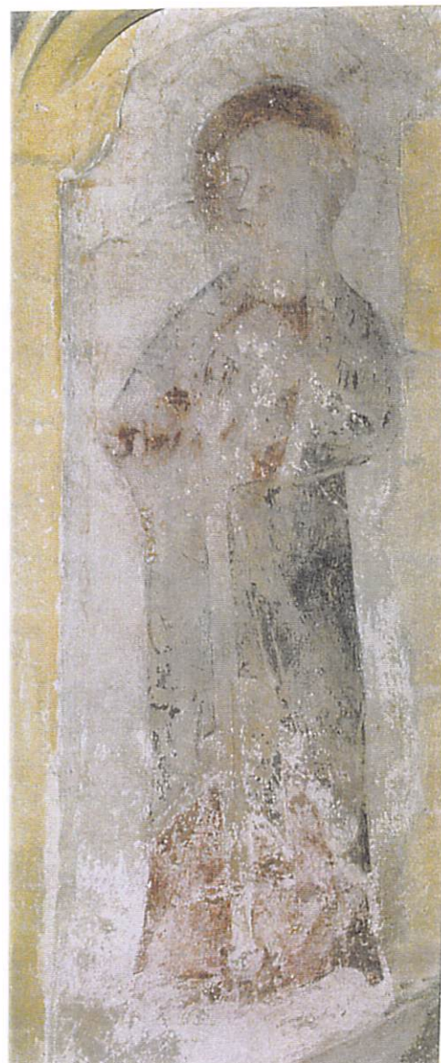
Plate 4. (Above left) General view of the north window on the west wall. (Photo: Tobit Curteis Associates 1997)
