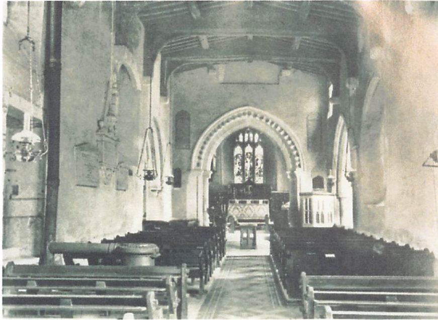
Fig 2. Church Interior looking East (Picture by Walton Adams & Sons. Reading )
