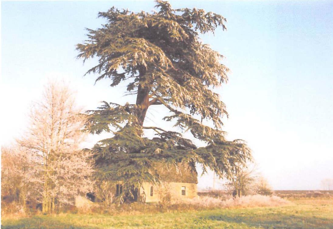
The Ivy Church on the south side of the main Cirencester to Fairford road. Services are still held here on various occasions.
